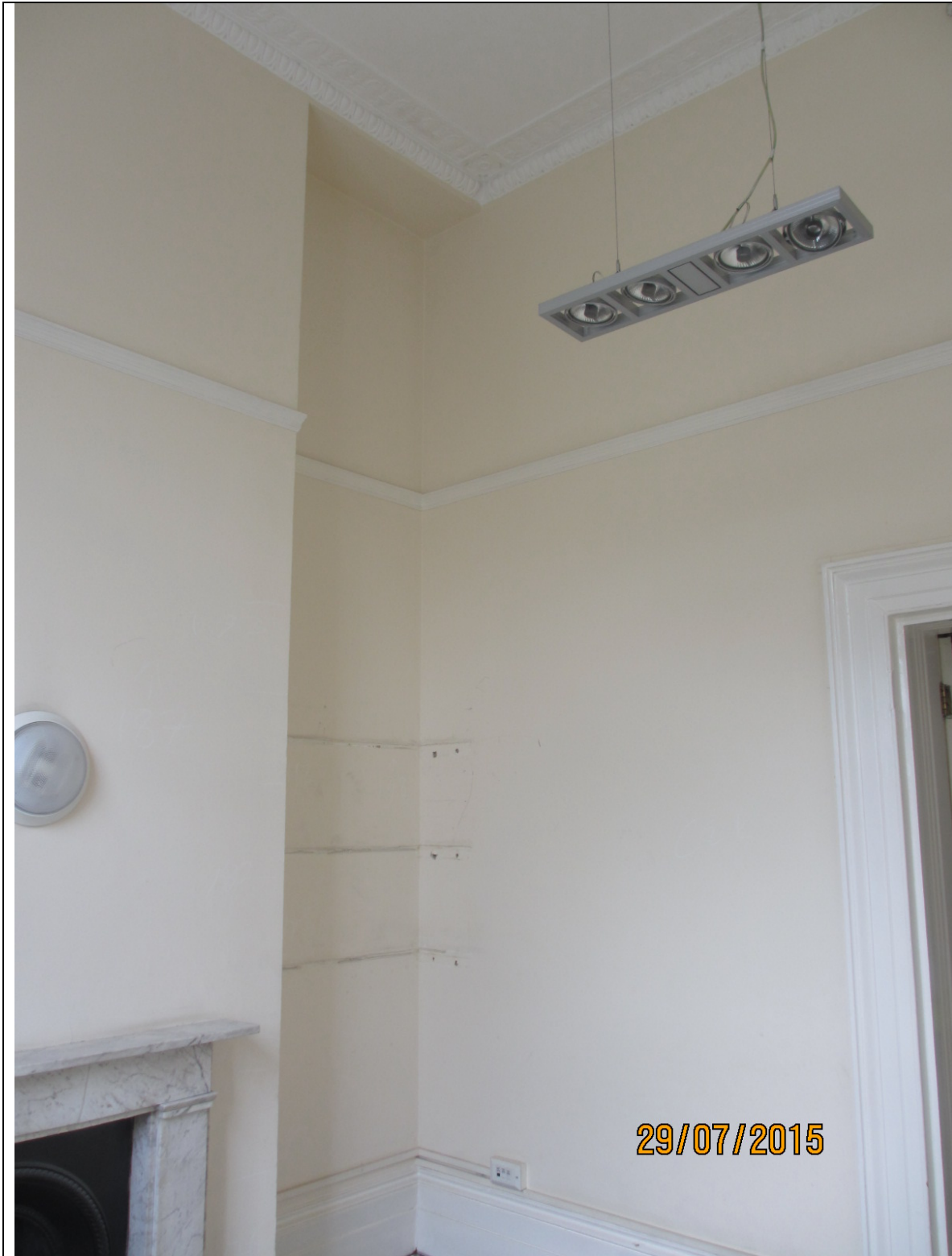
Photo 5: First Floor Garden Room to Lobby Wall (right hand wall) proposed for removal and cornice proposed to be concealed by elaborate suspended ceiling.
